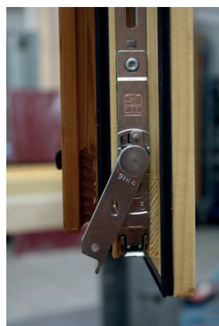
Fig. 1: Window sash of a composite scantling
